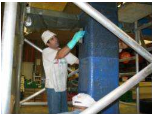
Application of Saturant on FRP Wrapping
