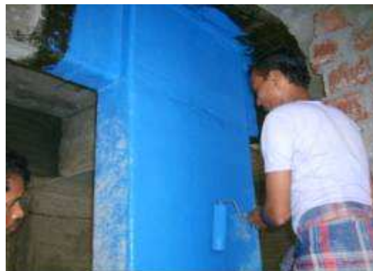
Application of Saturant on FRP Wrapping
