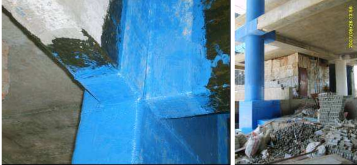
RC Columns after Completion of FRP Wrapping
