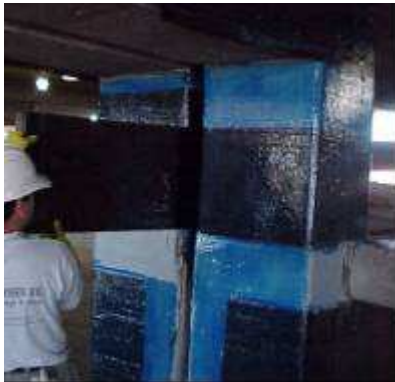
Wrapping with Carbon Fiber
