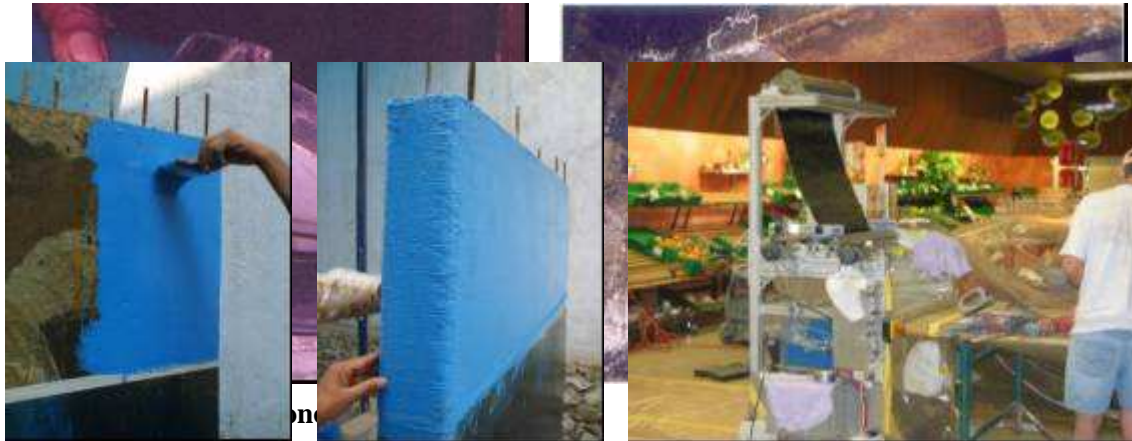
Application of Saturant
